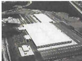
WalMart Distribution Center
